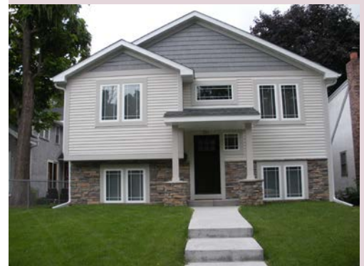
Single-Family Home, New Construction - 1st Ave S
