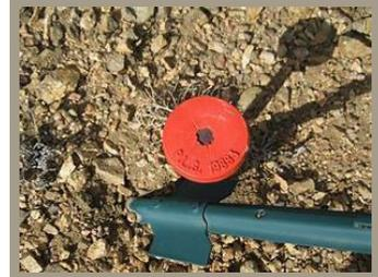
**Step 1.** Call Gopher State One at 811 or 651-454-0002 to locate utilities to ensure you can dig for the markers safely. Gopher State One should be contacted at least 48 hours before digging. This is a free service. Gopher State One contacts all the utilities and asks them to mark where their utility lines are on your property, so expect some paint marks.
